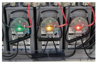
The IntelliBatt B-Nodes map to a battery automated reporting or BAR system which monitors the health of each battery and provides visual confirmation of battery status: Green = good; Yellow = trending; Red = maintenance required.
